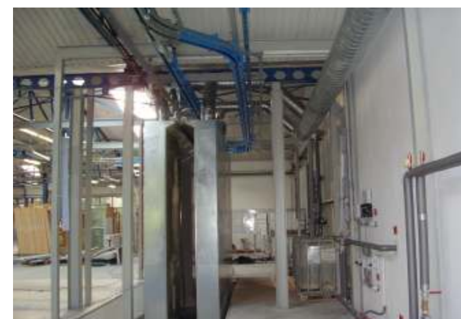
Flow-coat placeret i grav
